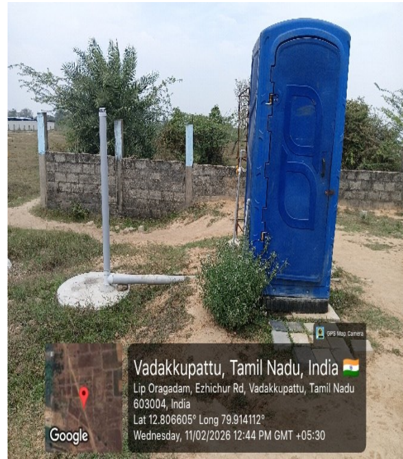
RESTROOM WITH SOAKPIT
