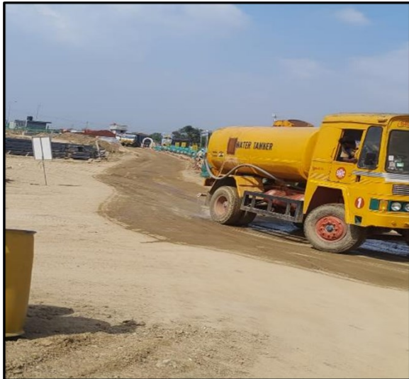
WATER TANKER- DUST SUPPRESSION
